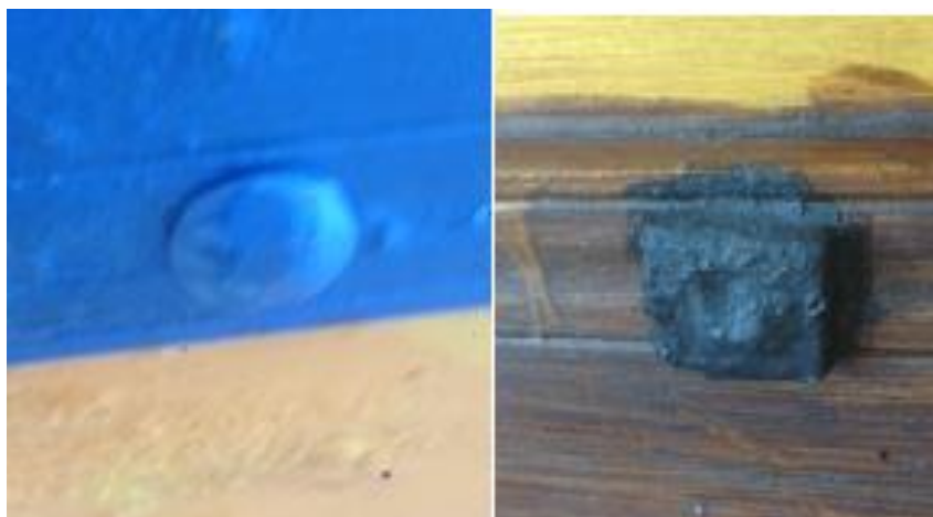
Figure 3: Example of bolts used in the reconstruction of the Dublinia's Skuldelev 2 ship.
